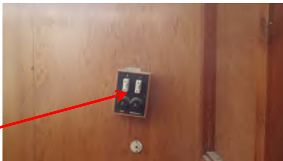
Photograph 15. Electrical backing board and fuse lining. 67 Platform, Multi-Purpose Hall (Visual Observation). Asbestos Presumed.
