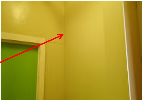
Photograph 27. Cement sheet walls. 88 Lobby, Multi Purpose Hall (Refer to 33538-125). Asbestos Presumed.
