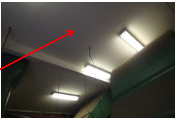
Photograph 23. Cement sheet ceiling. 79 PE Store, Multi Purpose Hall (Refer to 33538-129). Asbestos Detected.
