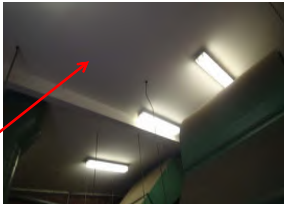
Photograph 21. Cement sheet ceiling. 76 & 77 Chair Store, Multi Purpose Hall (Refer to 33538-169). Asbestos Detected.
