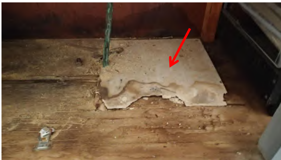
Photograph 2. Cement sheet debris, cupboard 33 Science, Science Wing (Refer to previous audit). Asbestos detected.
