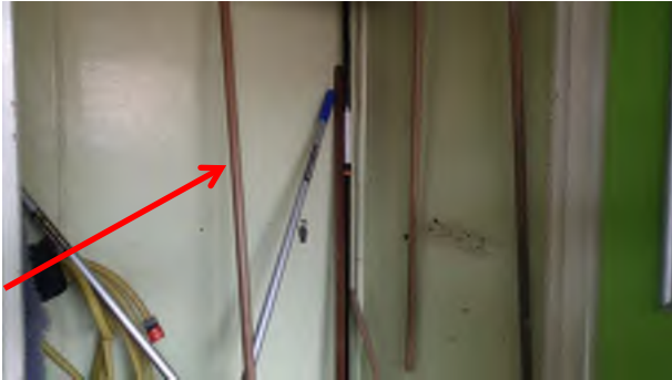
Photograph 19. Cement sheet walls. 71 CLNR, Multi Purpose Hall (Refer to 33538-160). Asbestos Detected.
