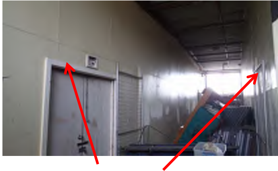
Photograph 7. Cement sheet walls. 64 Prop Store, Multi-Purpose Hall (Refer to 33538-147). Asbestos Detected.
