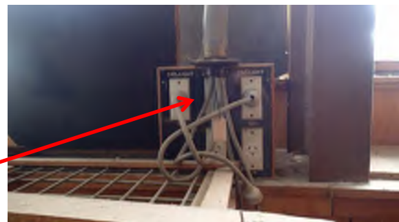
Photograph 30. Electrical backing board. 243 Store, Multi-purpose Hall (Visual Observation). Asbestos Presumed.
