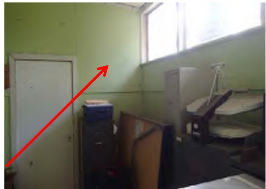
Photograph 28. Cement sheet walls. 91 Cloak, Multi Purpose Hall (Refer to 33538-110). Asbestos Detected.
