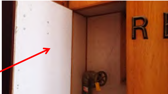
Photograph 25. Cement fire hose cupboard. 81 Hall, Multi Purpose Hall (Refer to 33538-158) Asbestos Detected.
