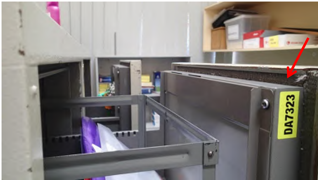
Photograph 4: Rope lining to filing cabinet. 57 Resource, Commerce Wing (DA7323) Asbestos detected.
