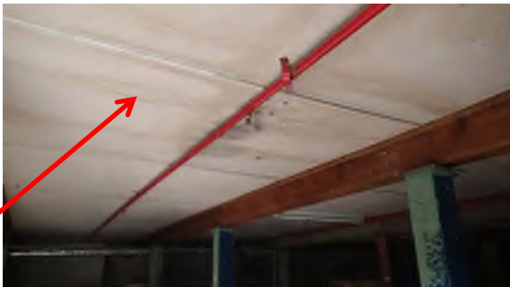
Photograph 35. Cement sheet eaves. External, Multi Purpose Hall (Visual Observation). Asbestos Presumed.
