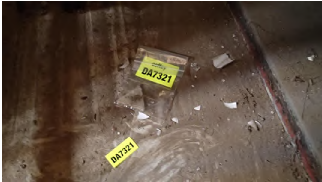
Photograph 3: Cement sheet debris. 264 Store, Commerce Wing (DA7321). Asbestos detected.
