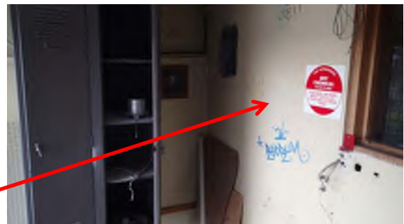
Photograph 18. Electrical backing board. 69 Steps (room Above), Multi Purpose Hall (Visual Observation). Asbestos Presumed.
