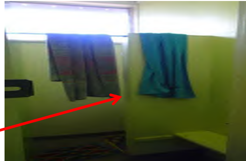
Photograph 28. Cement sheet walls. 91 Cloak, Multi Purpose Hall (Refer to 33538-110). Asbestos Detected.
