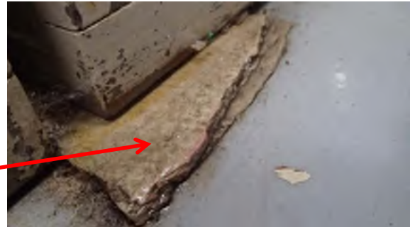
Photograph 4. Cement sheet debris. Commerce Wing, 264 Store (DA7321). Asbestos Detected.
