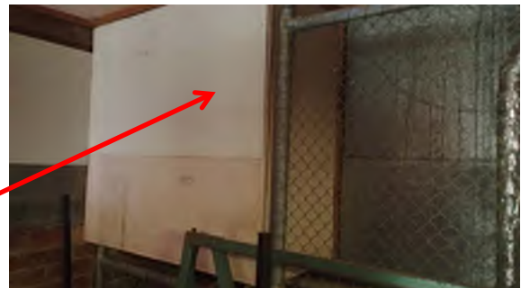
Photograph 36. Mastic wall expansion joint. External, Multi Purpose Hall (Refer to 33538-204). Asbestos Detected.
