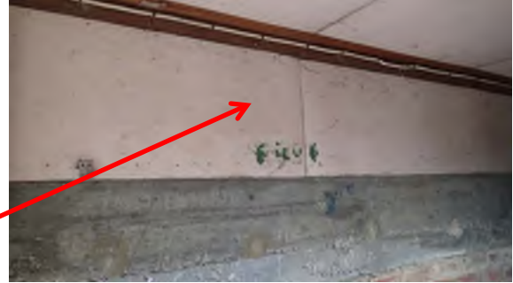
Photograph 34. Cement sheet partition walls. 244 Store (sub level below stage area), Multi Purpose Hall (Refer to 33538-180). Asbestos Detected.
