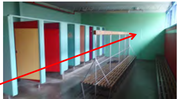
Photograph 10. Cement sheet walls. 66 Female Change, Multi Purpose Hall (Refer to 33538-162) Asbestos Detected.
