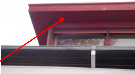
Photograph 5. Cement sheet clear storey eaves. External, Commerce Wing (Refer to 33538-270). Asbestos Detected.
