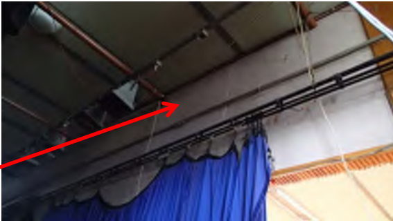
Photograph 13. Cement sheet infill panel. 67 Platform, Multi Purpose Hall (Refer to 33538-152). Asbestos Detected.
