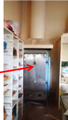
Photograph 44. Internal lining to kiln. 3 Clay Store, Trade Wing (Visual Observation). Asbestos Presumed.
