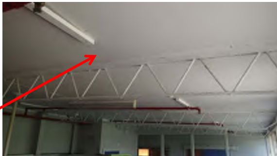
Photograph 9. Cement sheet ceiling. 65 Male Change, Multi Purpose Hall (Refer to 33538-139) Asbestos Detected.
