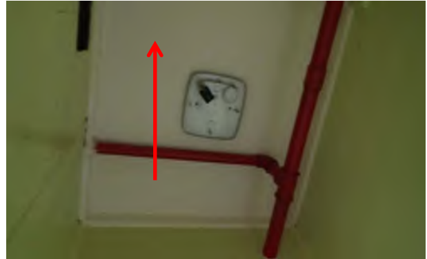
Photograph 20. Cement sheet ceiling. 71 CLNR, Multi Purpose Hall (Refer to 33538-161). Asbestos Detected.
