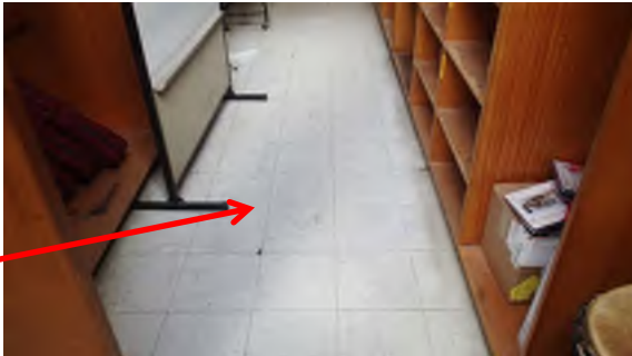
Photograph 39. Vinyl floor tiles. 103 Office, Music Block. (Refer to 33538-187x). Asbestos Detected.
