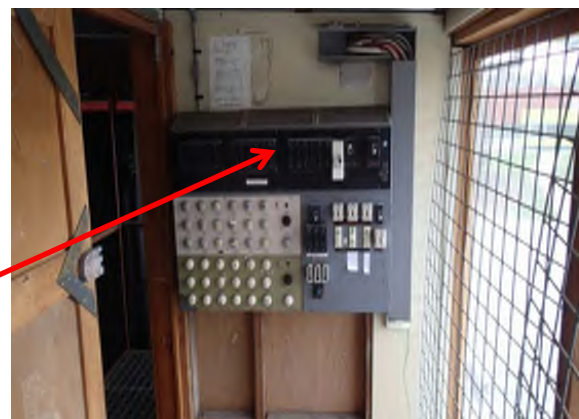
Photograph 18. Electrical backing board. 69 Steps (room Above), Multi Purpose Hall (Visual Observation). Asbestos Presumed.
