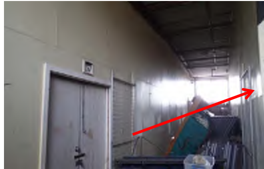
Photograph 16. Cement sheet walls. 69 Steps, Multi-Purpose Wing (Refer to 33538-155). Asbestos Detected
