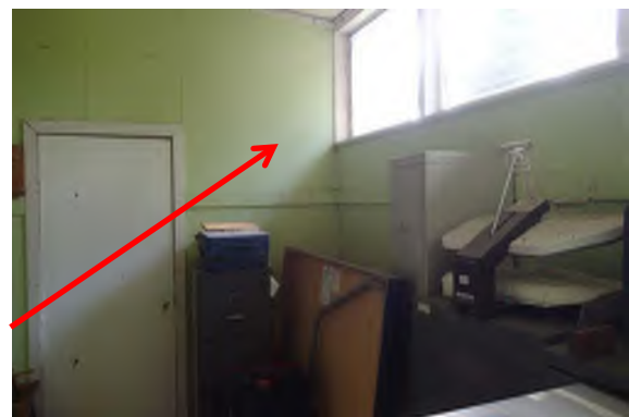
Photograph 24. Cement sheet walls. 80 PE Store, Multi Purpose Hall (Refer to 33538-170). Asbestos Detected.
