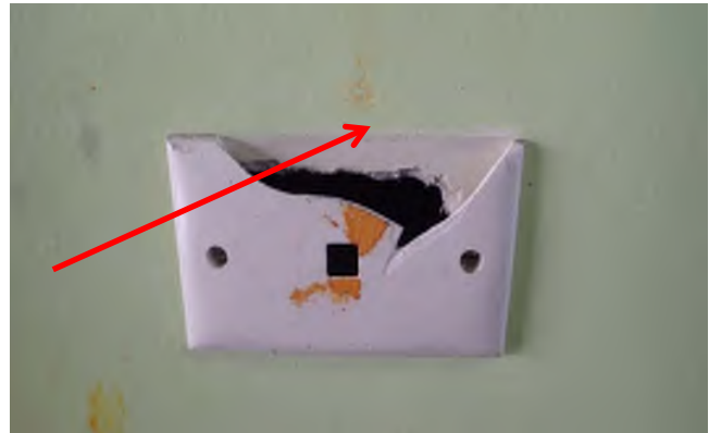
Photograph 22. Cement sheet walls. 79 PE Store, Multi Purpose Hall (Refer to 33538-128). Asbestos Detected.
