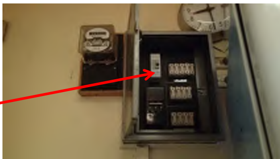
Photograph 29. Electrical backing board. 93 Servery, Multi Purpose Hall (Visual Observation). Asbestos Presumed.
