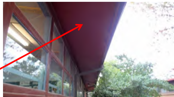
Photograph 6. Cement sheet eaves. External, Commerce Wing (Refer to 33538-275). Asbestos Detected.
